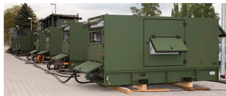
Parallel operation AVS 40 kW VSCF Genset
