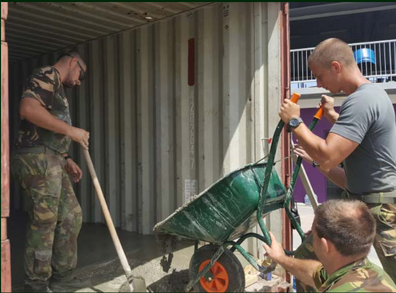
Betonstorten in douchecontainer noodhuisvestingsproject Festival Village
